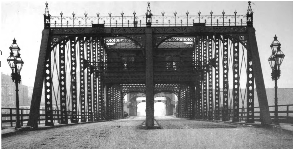
Above, two views of a typical Chicago Bridge viaduct in 1888, note that this structure is completely separate and before the connection to the actual bridge span. These funneled pedestrians and vehicles in an orderly manner onto the bridge, where policemen were stationed to close the street when the bridge was to be opened. At right, the “municipal device,” an example of the type of ornamentation included on such bridge work. Below, the new bridge, also designed by Roemheld, that replaced the 1888 bridge 18 years later
