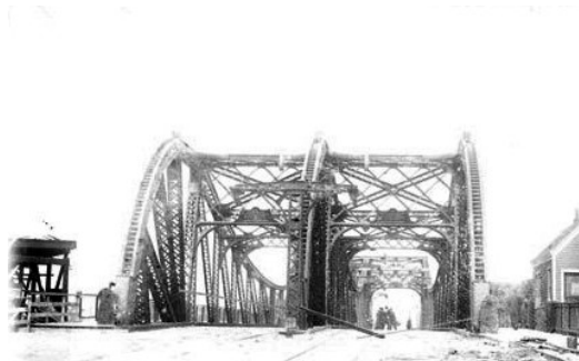
Two of the prominent and historical bridges designed by Roemheld following break out with his own company: the North Halsted Street Bridge, built in 1909, and the West Division Street Bridge, built in 1903 - one of the oldest surviving functional bascule bridges in North America.
